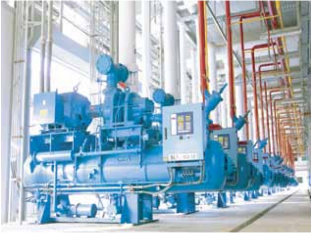
Photo 1 : 46 sets and 18,000 HP of Screw Compressor.
