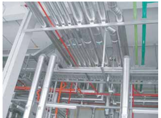
Photo 4 : Piping Installation with Stainless Steel Cladding.
