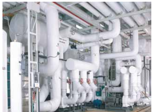
Photo 6 : Vessel and White Preform PVC Cladding.
