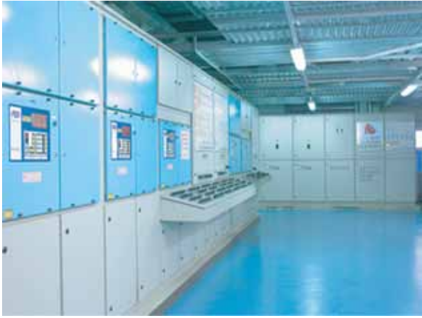
Photo 7 : Micro Processor Remote Monitoring Control & Mimic diagram.
