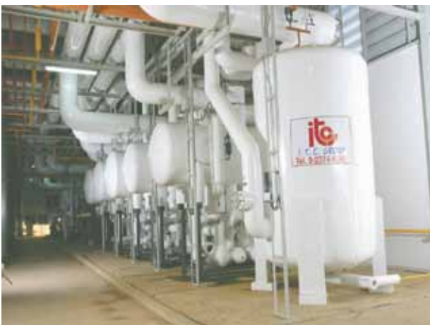
Photo 5 : Pump packaged with PU-Insulation.
