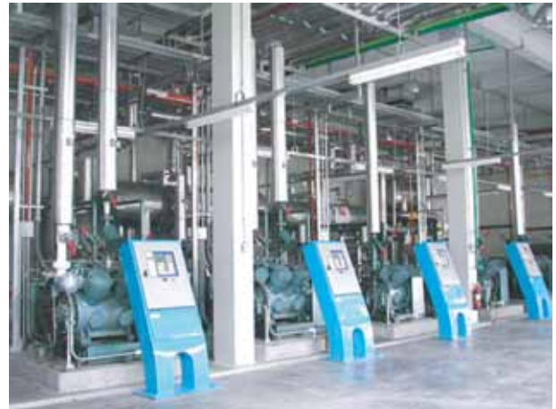
Photo 2 : Reciprocating Compressor with Microprocessor Control.
