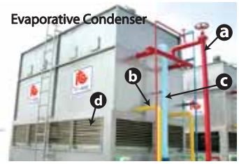
Figure 1-Evaporative Condenser a) Red pipes indicates hot vapor gas. b) Yellow pipes indicates the condensed liquid refrigerant. c) Blue pipes containing water to recirculate for heat exchange. d) Air inlet allows air inside for heat exchange.
